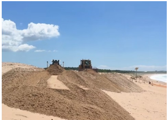
Earthmoving equipment will reshape the dune.
