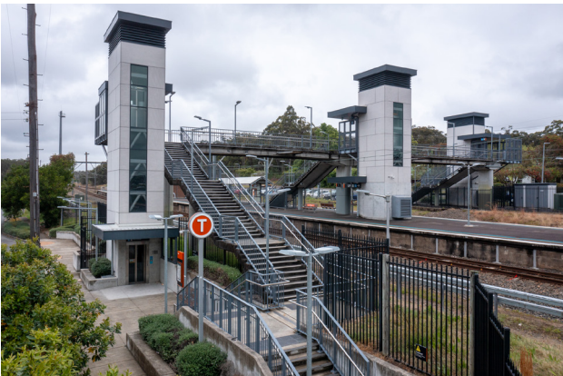
Wyee Train Station
