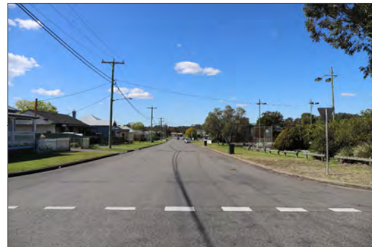
View H2 - Views north, south, east and west within the commercial axis
