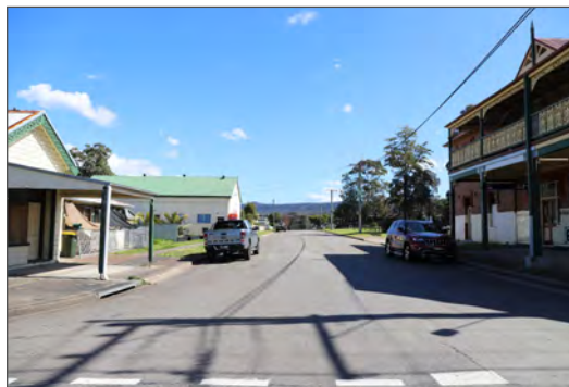
View H2 - Views north, south, east and west within the commercial axis
