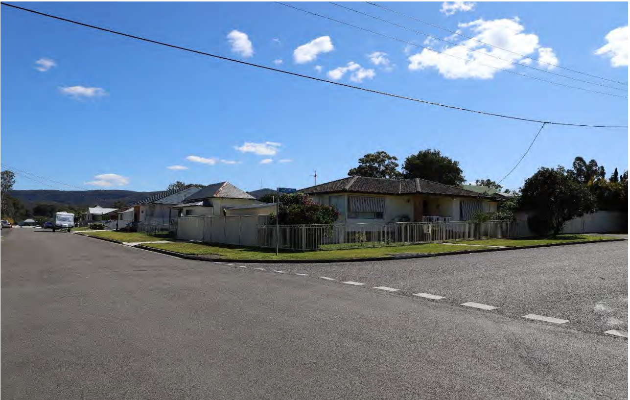
Plate 7.10 View facing northwest across the current 10 metre height limit building zone
