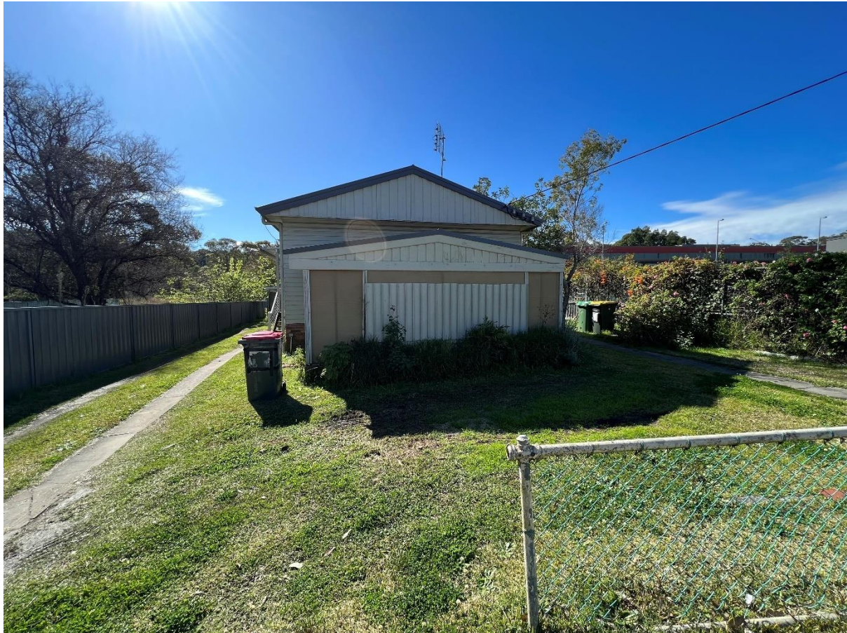
Figure 6c. Street side view, facing north, of the main structure currently on the Site. Two concrete paths on either side of the house and an old chain link fence can also be seen. Photo taken 17 Aug 2023.
