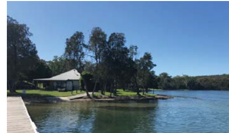
Image 5 JetBuzz watersports building viewed from the jetty
