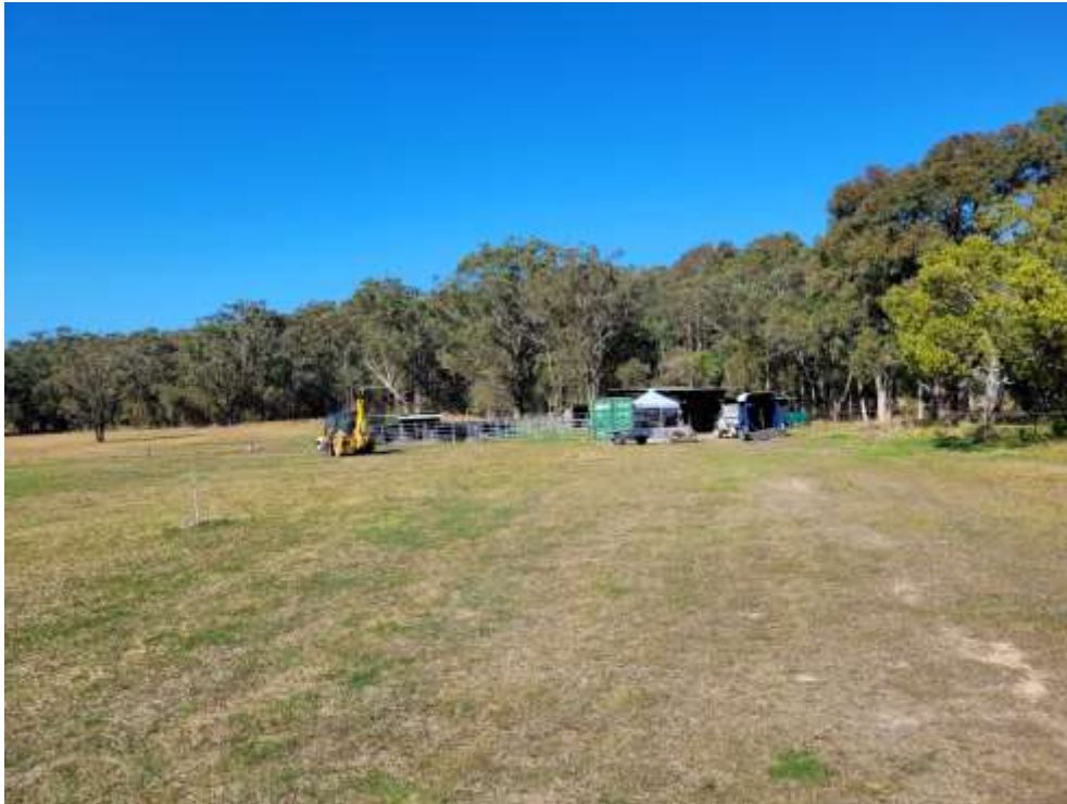
Horse stables at the central-western portion of the site with containers and sheds.
